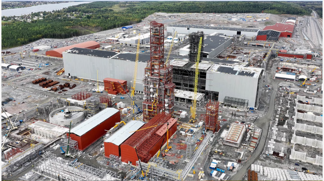
Stegra construction site
