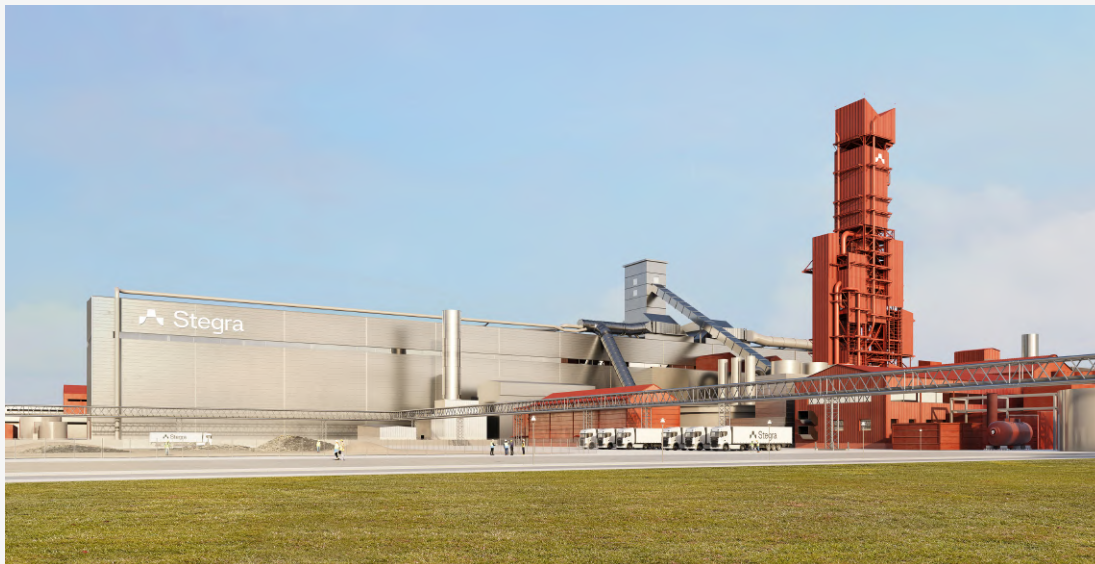
An artist's rendering of the Stegra steel plant under construction in Sweden.
