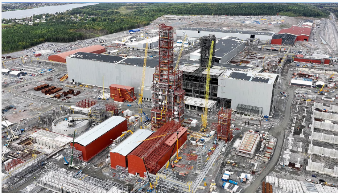
Stegra construction site
