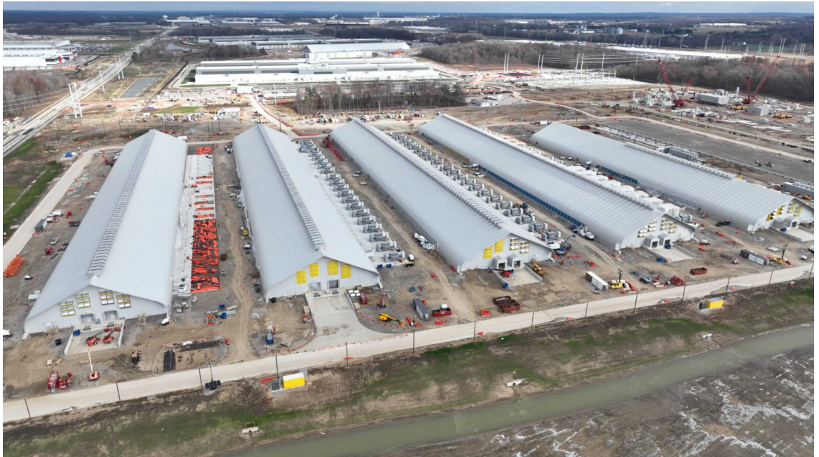
Meta, the parent company of Facebook and WhatsApp, has put AI data centres into huge tents in Ohio, a sign of the feverish construction boom as technology companies race each other to capture the market. They are making enormous demands for land, electricity and water.
